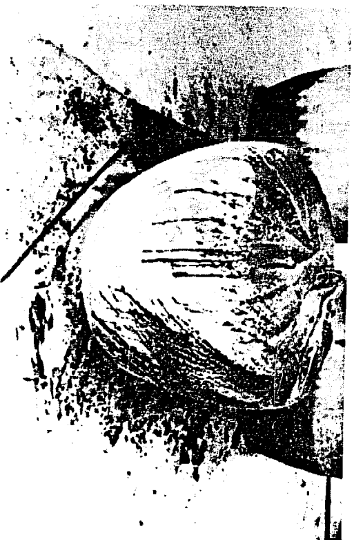
2.6 Spray some water on the mould before plastering to make it damp.
